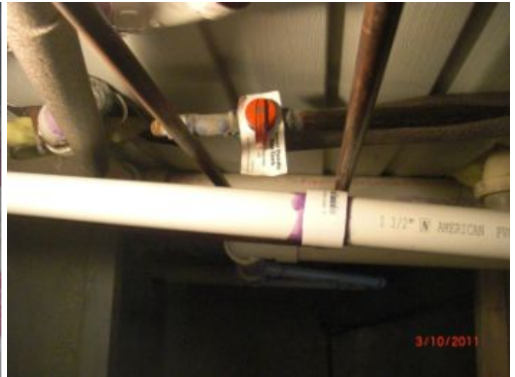
Gas shut off valve located in the basement
