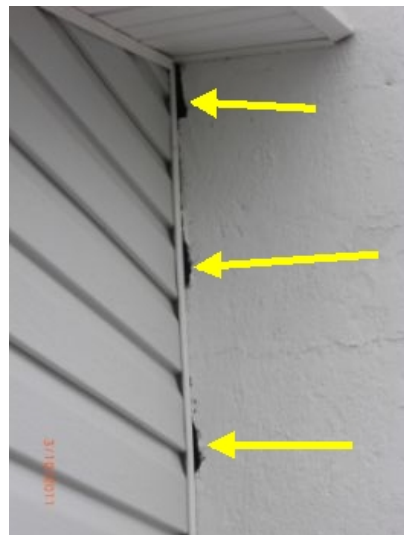
Evidence that chimney is leaning away from house.
