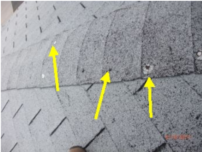
Evidence of roof repair (shingle are nailed on lower section)
