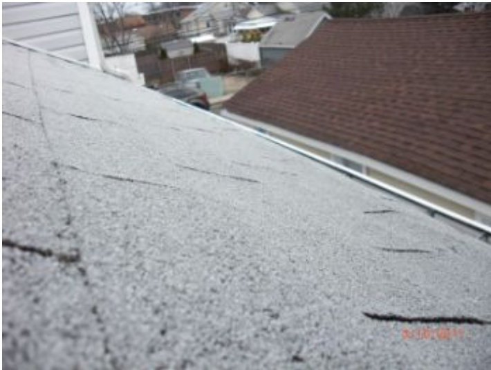
Roof is wavy at the back of the house
