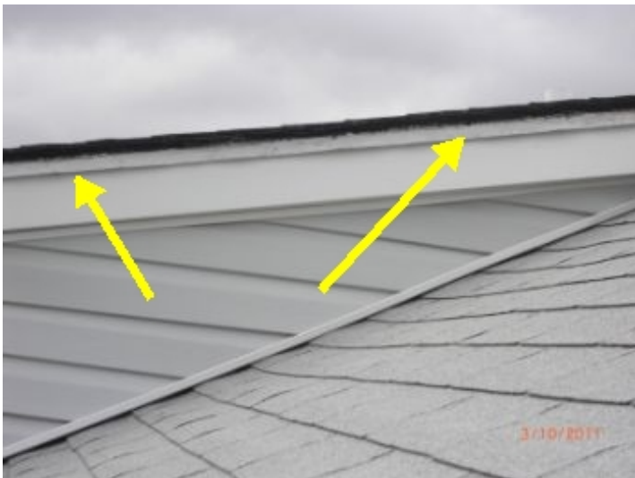
Peeling paint, needs to be scraped and painted
