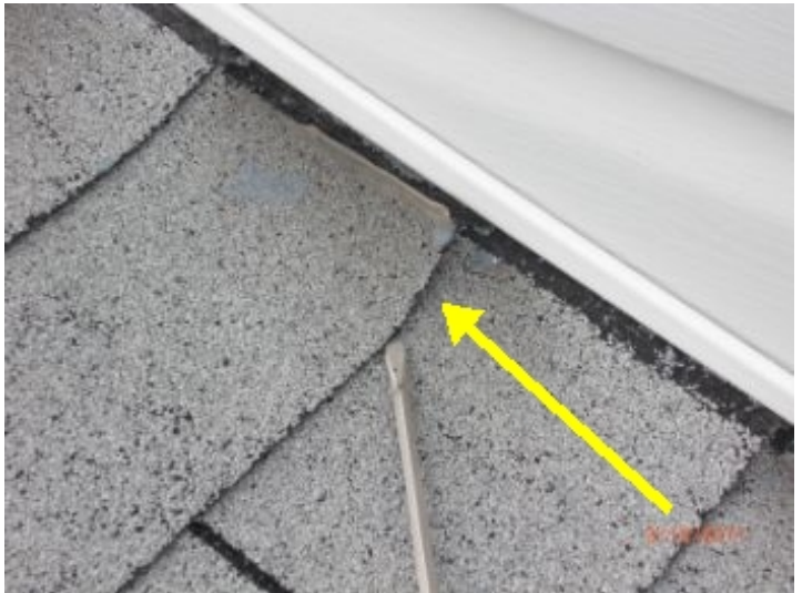
Shingles are peeling up. This was located on the front shed roof.
