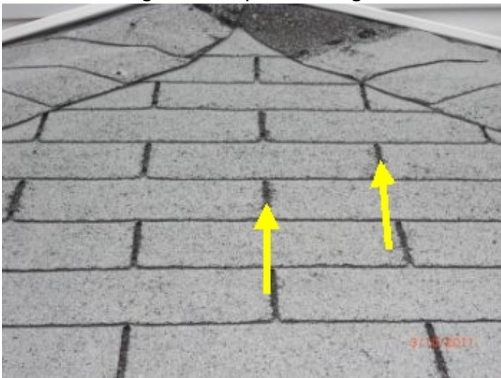
spacing between roofing shingles suggests roof is getting towards the end of its useful life
