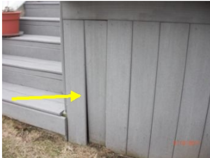
Loose side board on deck
