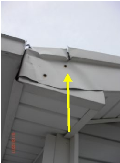
Cracked/ ripped trim at the rear of house
