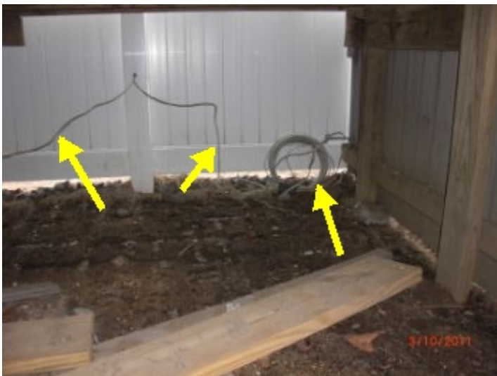
loose wire for outdoor lighting under deck
