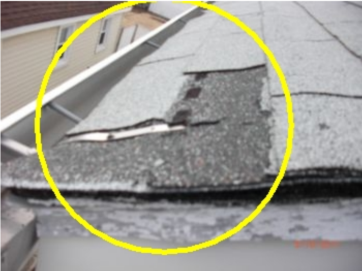
missing shingles on front shed roof
