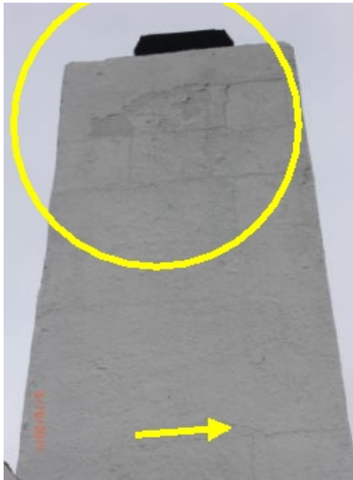
Cracking and peeling paint present on chimney
