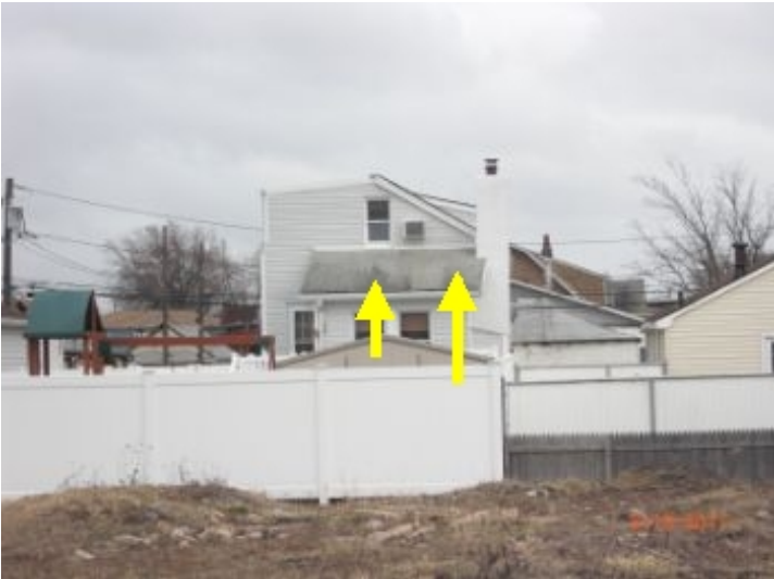
Algae staining is present on the rear part of the roof
