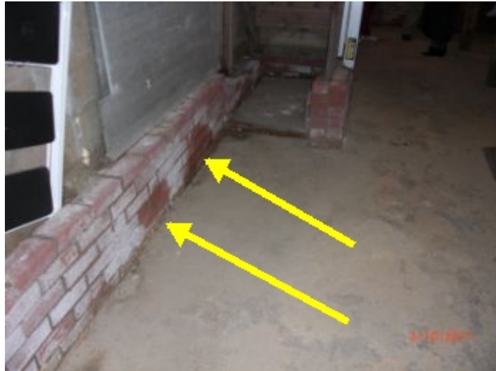
evidence of past flooding in basement
