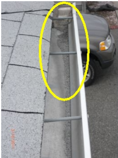
Roof granule is present in gutters
