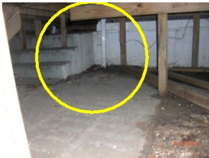
Gutter downspout terminates under the rear deck - suggest adding an extension to move waterflow away from foundation
