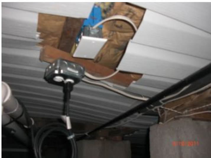
Basement outlets should be GFCI
