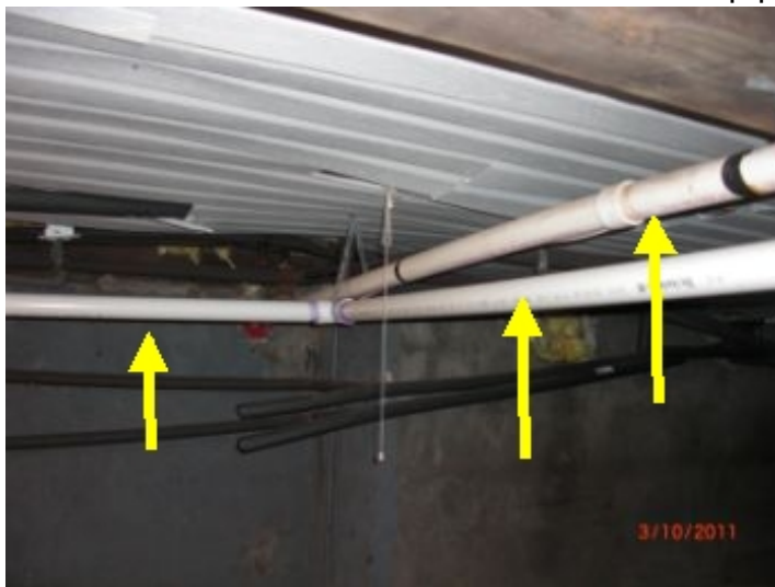
pipes for sump pump
