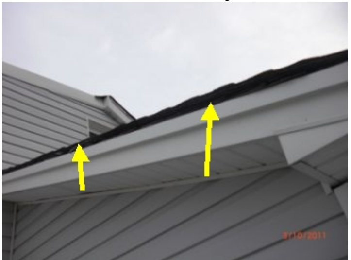
Multiple layers are present on the back part of the roof
