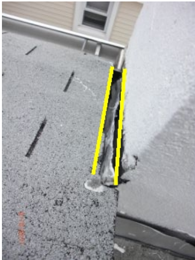
Improper flashing at roof and chimney resulting in a gap between roof and chimney
