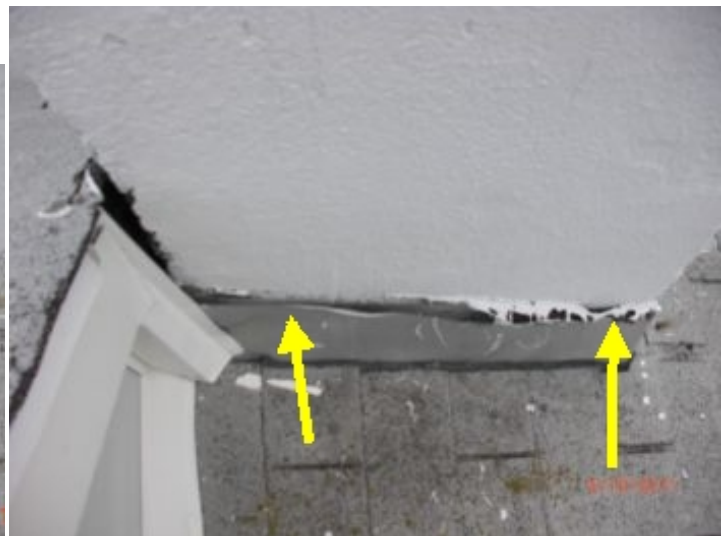
Improper flashing at roof and chimney
