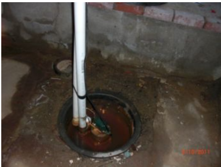
Basement sump pump - Rear location
