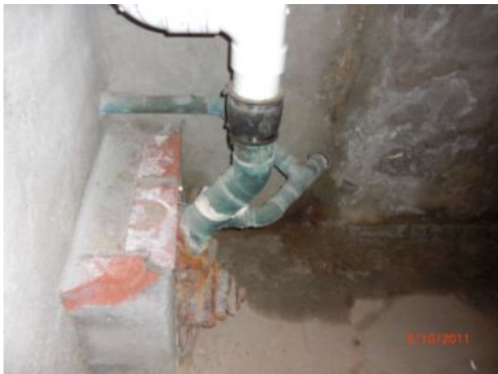
Main drain stack, located on the north rear side of the basement
