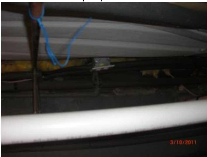
Outlets in basement should be GFCI due to flooding
