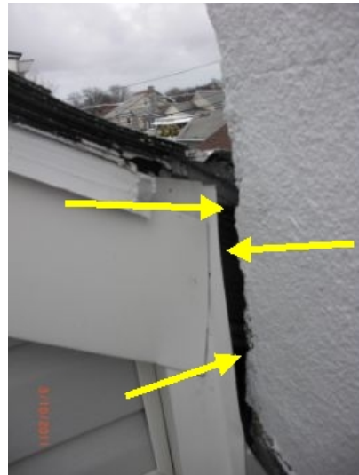
gap between chimney and house
