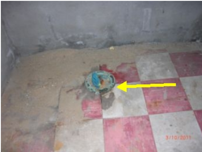
old flange for what appears to be a toilet in the basement
