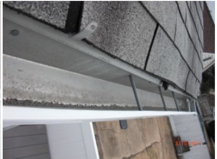
roof granules in gutter
