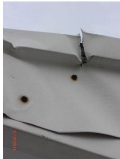
cracked/ ripped trim at rear of house
