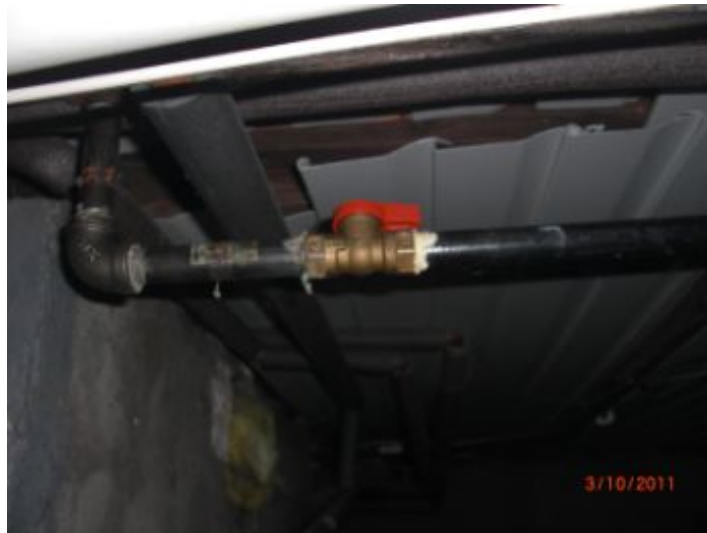
gas shut off valve
