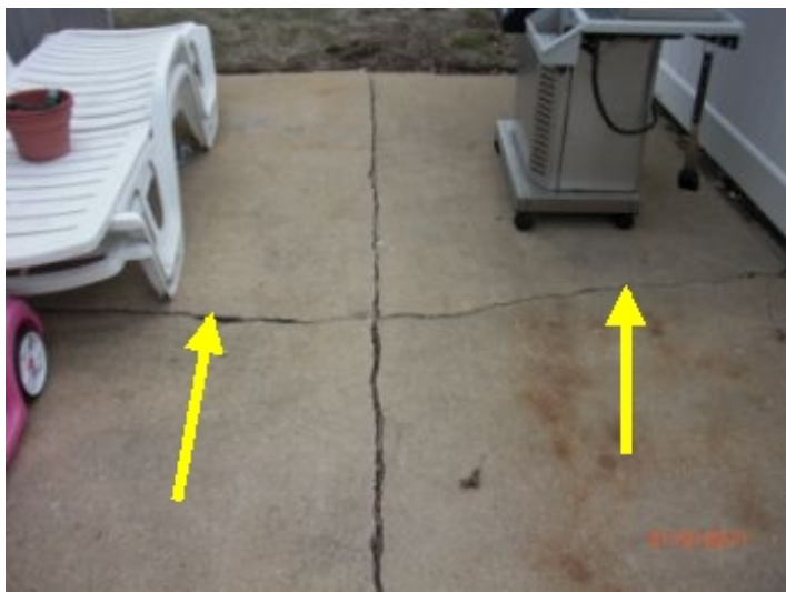
Minor cracks in rear patio
