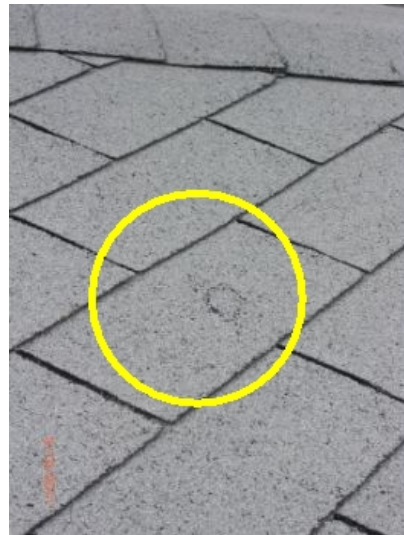
cracks in roof shingles
