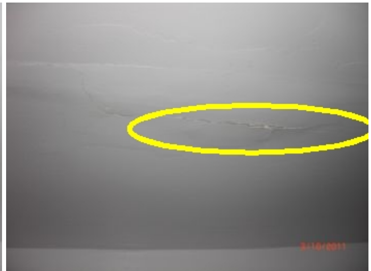
Moisture meter indicates that there is moisture present in this area
