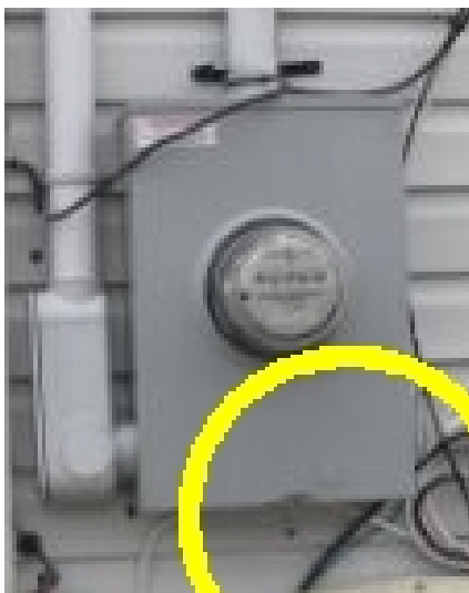
Electrical meter missing locking tab
