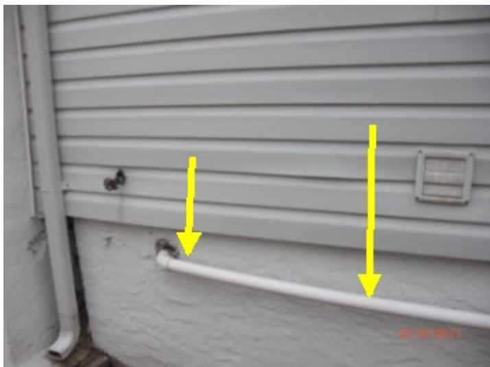
Sump pump over flow line
