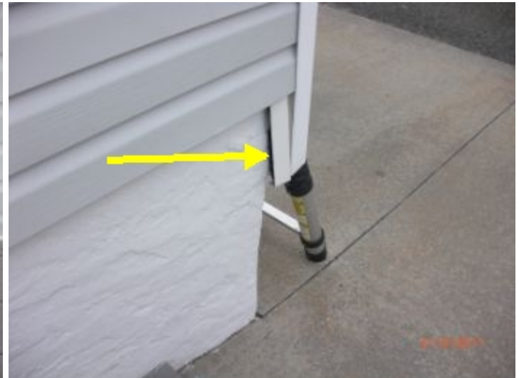
trim is cracked and pulling away from house (front corner by driveway)
