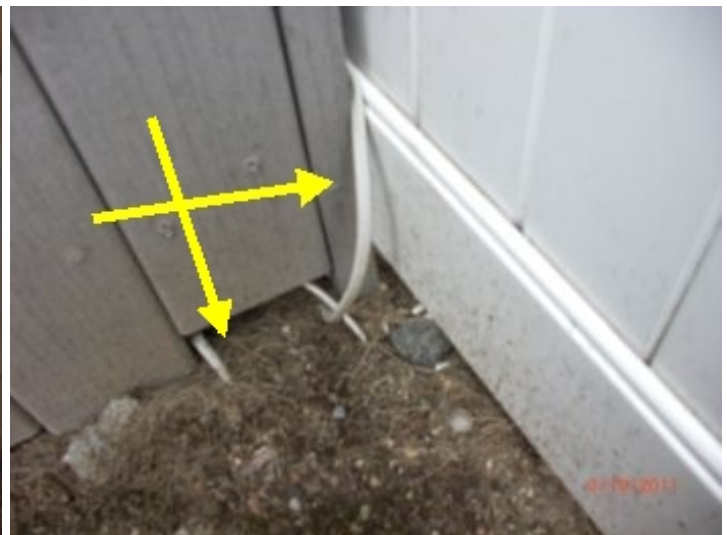
loose un buried wire for outdoor lights
